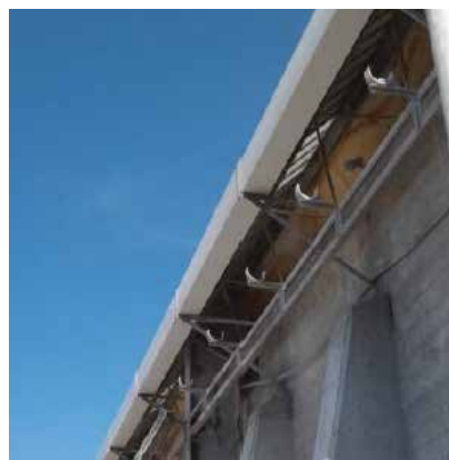
New spouting for better site water control.
