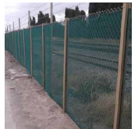
New screening near site intake system.
