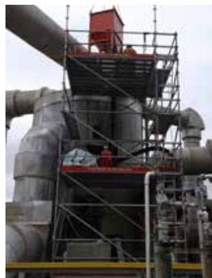
Catalyst replacement at Acid Plant
